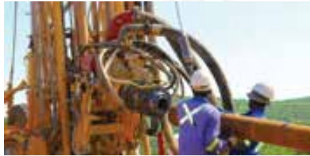
Borehole drilling process: technical workers replace drilling rod.
