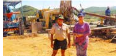
At the borehole drilling site: City of Windhoek's Ms. Zelda Scheepers, and Prinsloo Drilling site manager.
